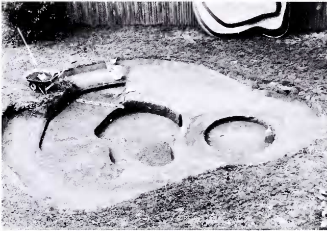
Figure 4. View of excavation for wetland complex in September 1985
